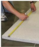
Start at a square corner of the room. Measure length and width of blanket needed saw equipped with a for wall application. Then measure and mark blanket.
